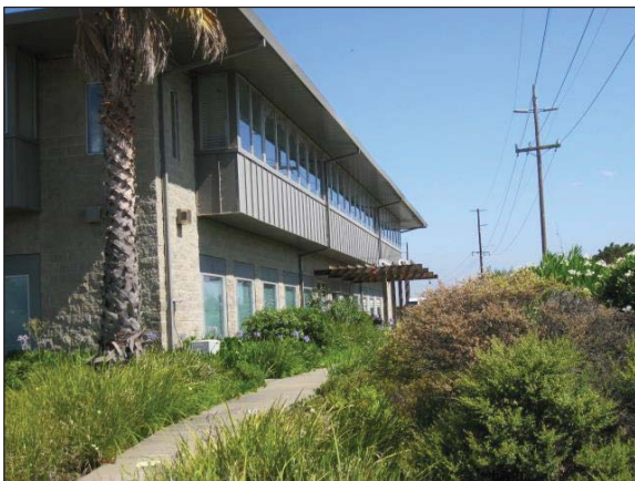
Rear View (eastern elevation)
