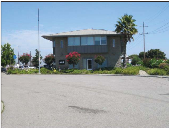
Side View (southern elevation) and Entrance to Parking
