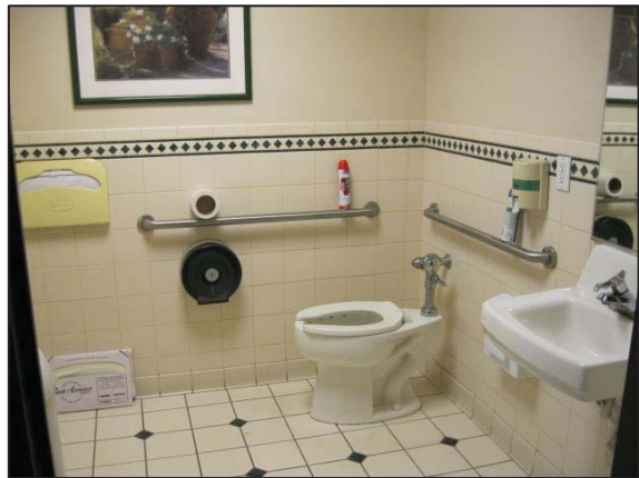
1 st Floor Common Area Restroom
