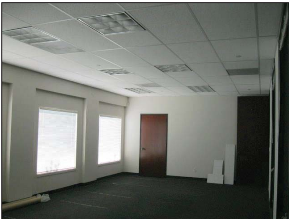
Vacant 1 st Floor Space
