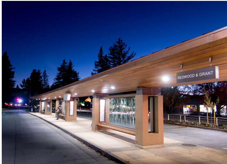
Figure 2 – Redwood Blvd & Grant Ave completed in 2017
