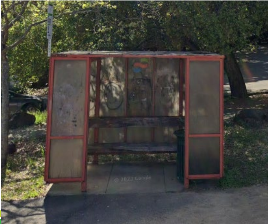
Example Shelter in GGBHTD Transfer Request
