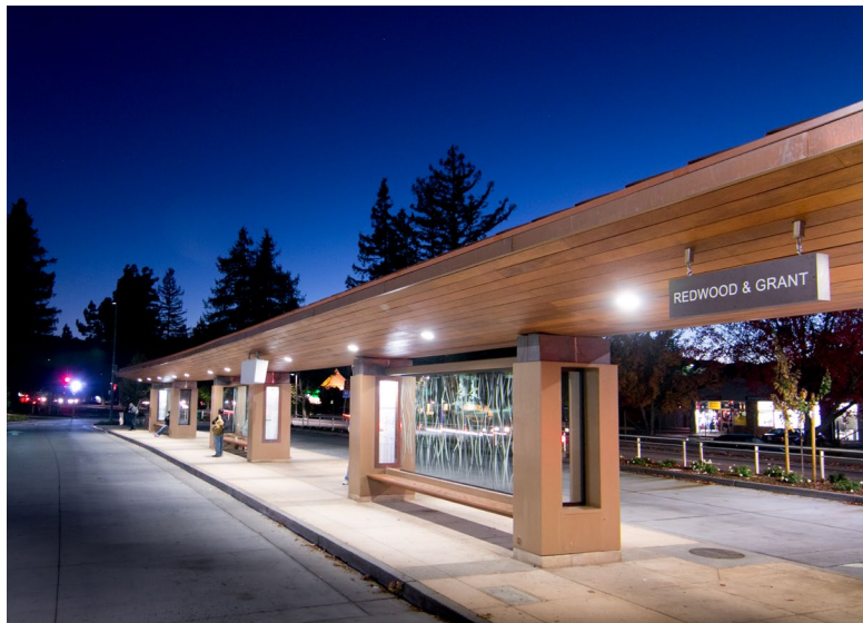
Figure 1 – Redwood Blvd & Grant Ave completed in 2017
